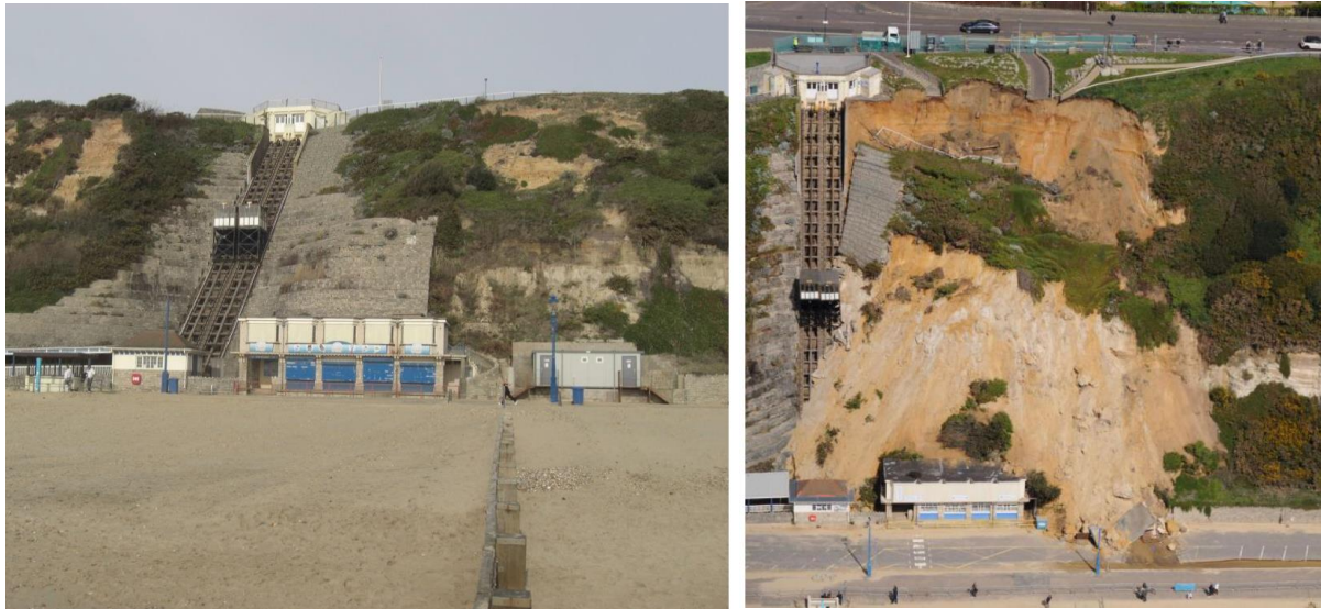
Figure 6 Before and after photographs of the East Cliff Lift slip in 2016 (images courtesy of Andrew Emery, 2016).
